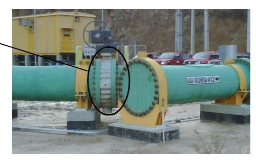
The applicable tool for the flanges specified is the ZGFSTE fitted with M48  $1^{7}/_{8}$ " collets.
